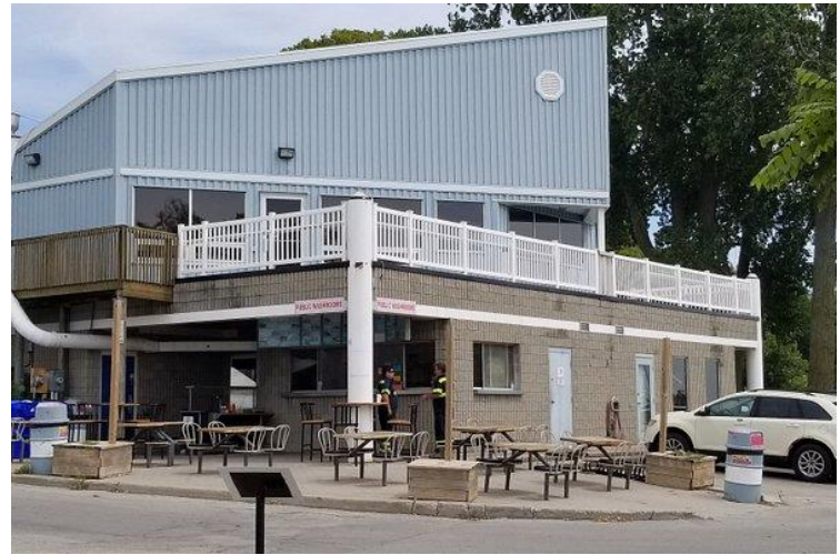
Figure 9: Colchester Community Centre (Source: Town of Essex)
