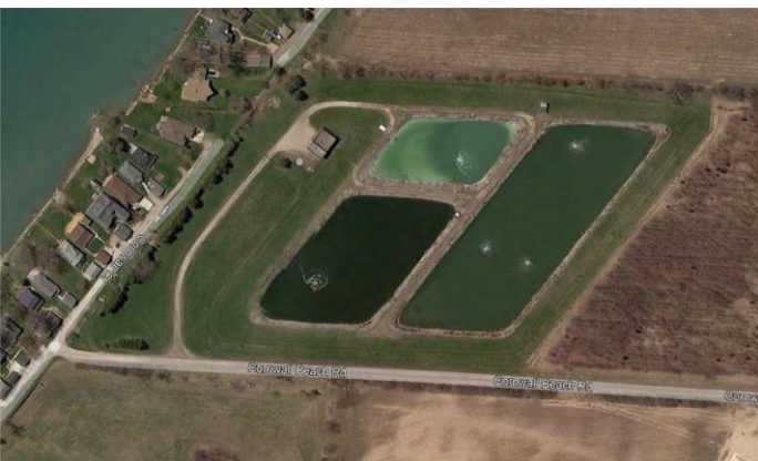
Figure 7: Colchester South Wastewater Treatment Facility (Source: Google Earth)
